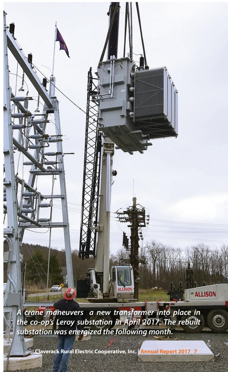
A crane maneuvers a new transformer into place in the co-op's Leroy substation in April 2017. The rebuilt substation was energized the following month.
