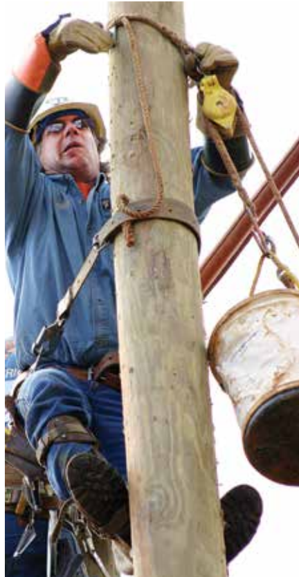
BACK IN THE DAY: Wysox Crew Chief Lindsay Chamberlain works atop a pole in 2005, when most electric lineworkers climbed poles using just the gaffs attached to their boots and their hands. Once they reached the work area, a leather safety strap would be wrapped around the pole to hold them in place and free their hands. Today, lineworkers must wear a protective device called a wood pole fall restraint when climbing and working on poles. It's one of the many changes Chamberlain has seen during his 36 years with the cooperative.
