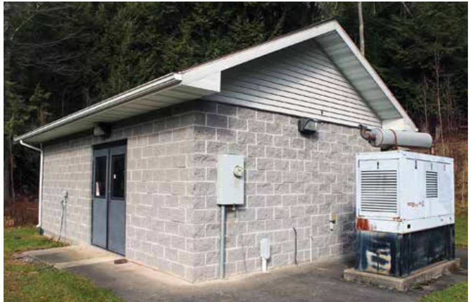
CO-OP POWERED: The Towanda Municipal Authority's chlorination building at Eilenberger Springs in Albany Township has been powered by Claverack since it was constructed in 1996. The underground springs on the authority's 25-acre property supply water to the boroughs of Towanda, Monroe, and New Albany, as well as portions of North Towanda, Towanda, and Wysox townships.
